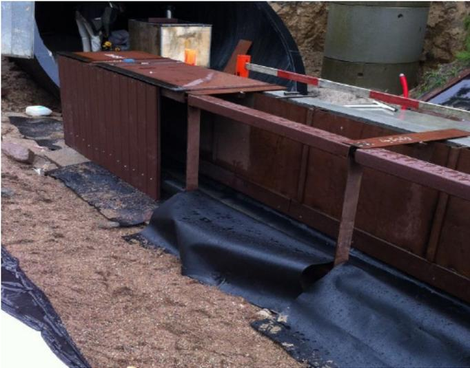
The upper part of the Environmental Bullet Catcher is covered with steel lids with overlap. The lids are mounted on fixed spacers and hinged to the rear edge of the concrete wall. The lids have a slight drop towards the concrete wall. In front of all lid and middle pieces, there is an edge steel "knife" that guides projectiles down into the box. On the underside of the lid and middle pieces, there is a projectile rear stop.
